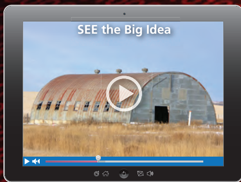
Quonset Hut (p. 174)
