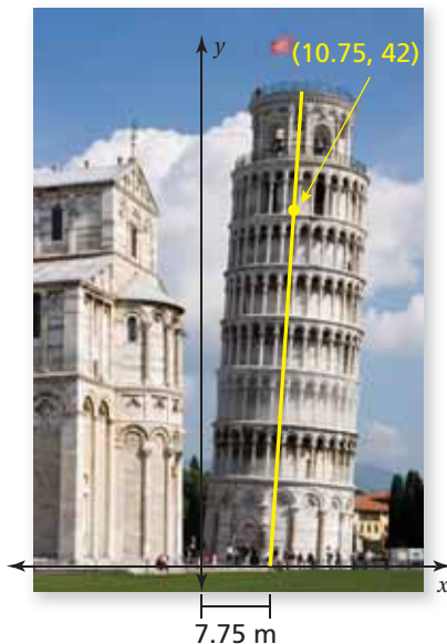
Leaning Tower of Pisa
