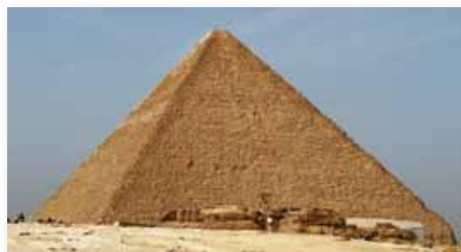
Cheops Pyramid in Egypt Height: about 480 ft Base: about 755 ft by 755 ft
